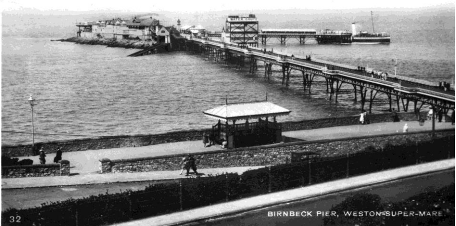
Fig. 2. Birnbeck Island, Pier and jetty, c1930
