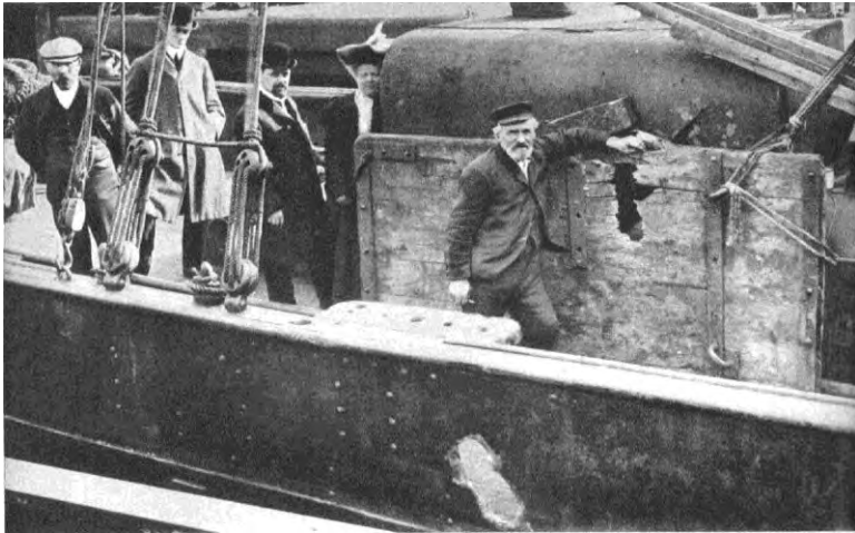
Fig.1: One of the damaged trawlers
