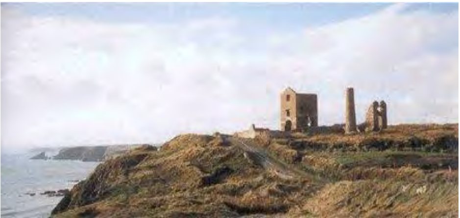
Fig. 12. Partly restored engine house at Knockmahon looking west towards Bunmahon (22) .
