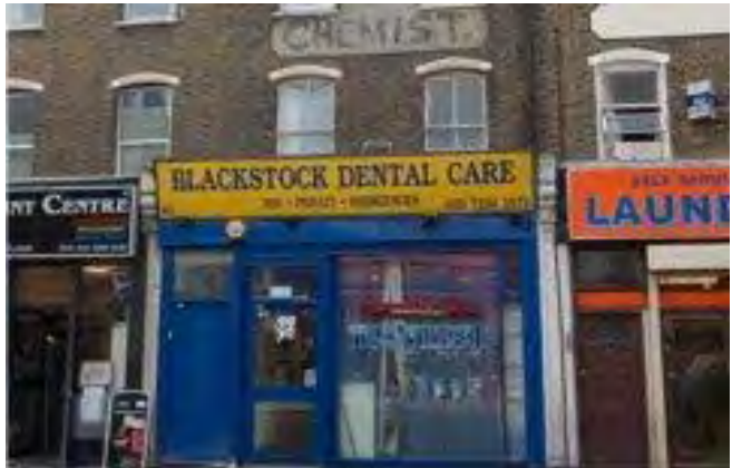
Fig. 2. Shopfront at 60 Blackstock Road.
