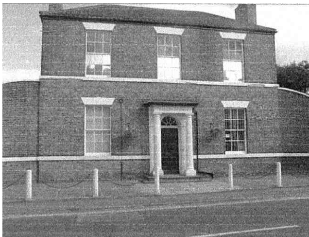
Fig.2: Easterfield House, Driffield
