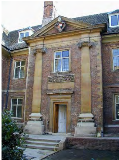
Fig. 3. Recent photograph of entrance Bishop's Hostel.
