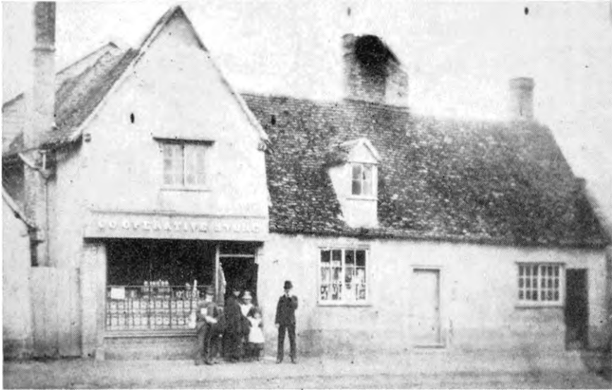
Fig. 1. Sawston co-operative Store c.1880 (3) .
