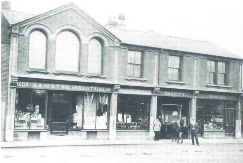
Fig. 3. Sawston Industrial & Co-operative Society Store c.1900 (7) .
