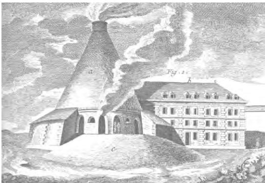
Fig. 3. Mid 18 th century English glass house with external furnace (10) .
